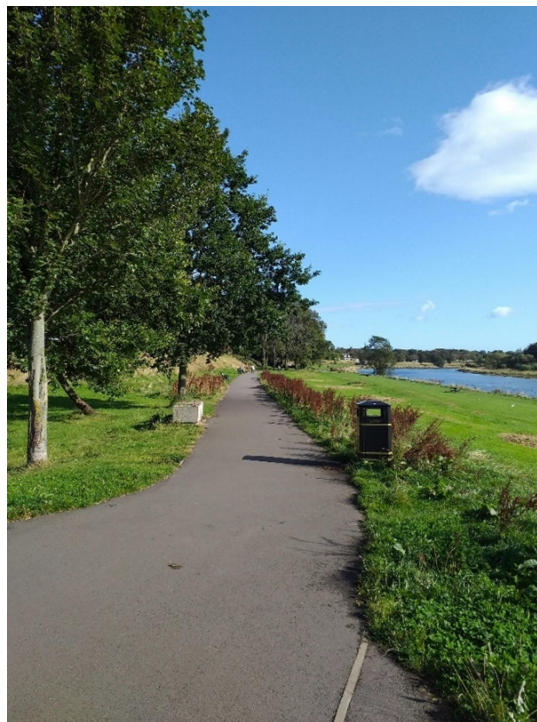
Figure 3-13 - Current Condition of the Eastern Section of the Riverside Path
